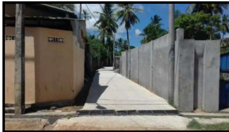
Photo of after the completion
