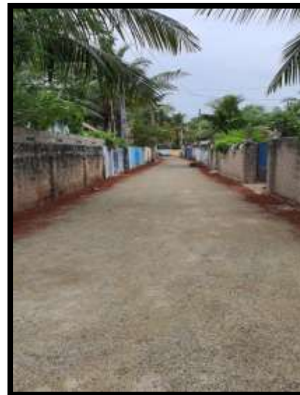
Photo of after the completion
