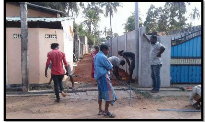
Photo of ongoing
