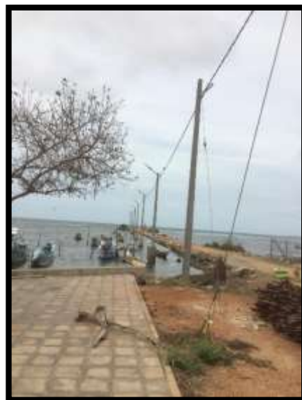
Photo of after the completion
