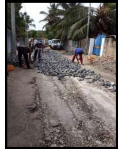
Photo of ongoing
