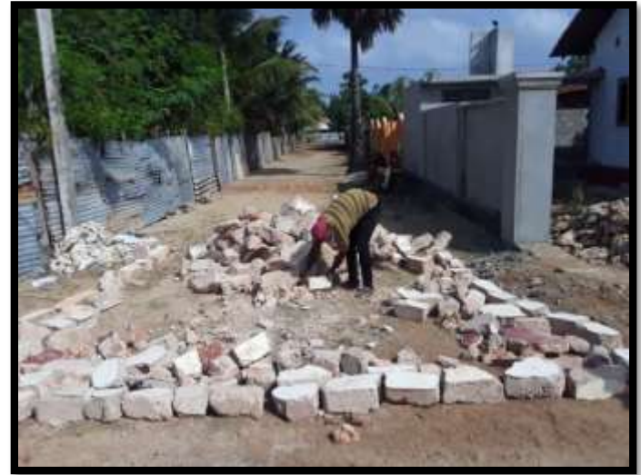
Photo of after the completion
