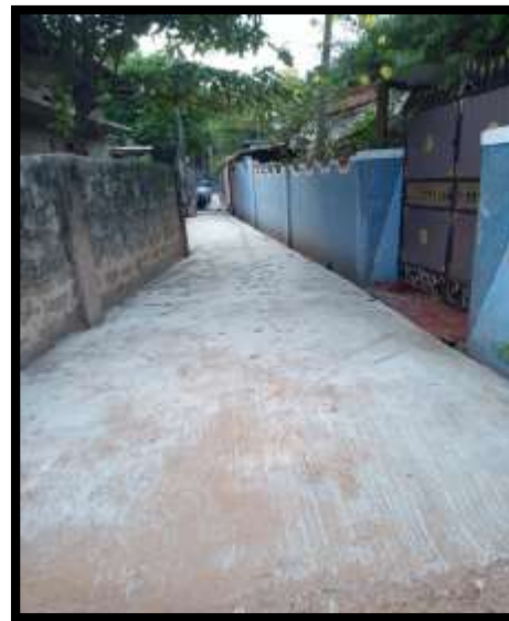
Photo of after the completion
