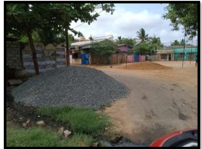
Photo of ongoing
