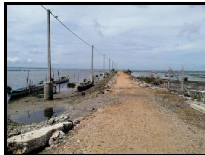
Photo of ongoing
