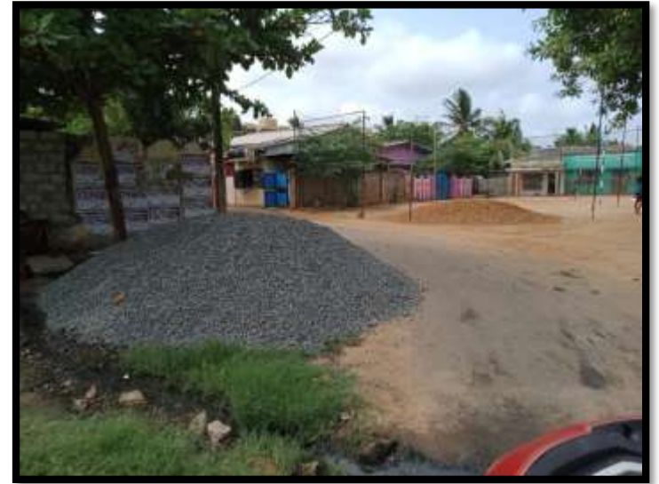
Photo of ongoing
